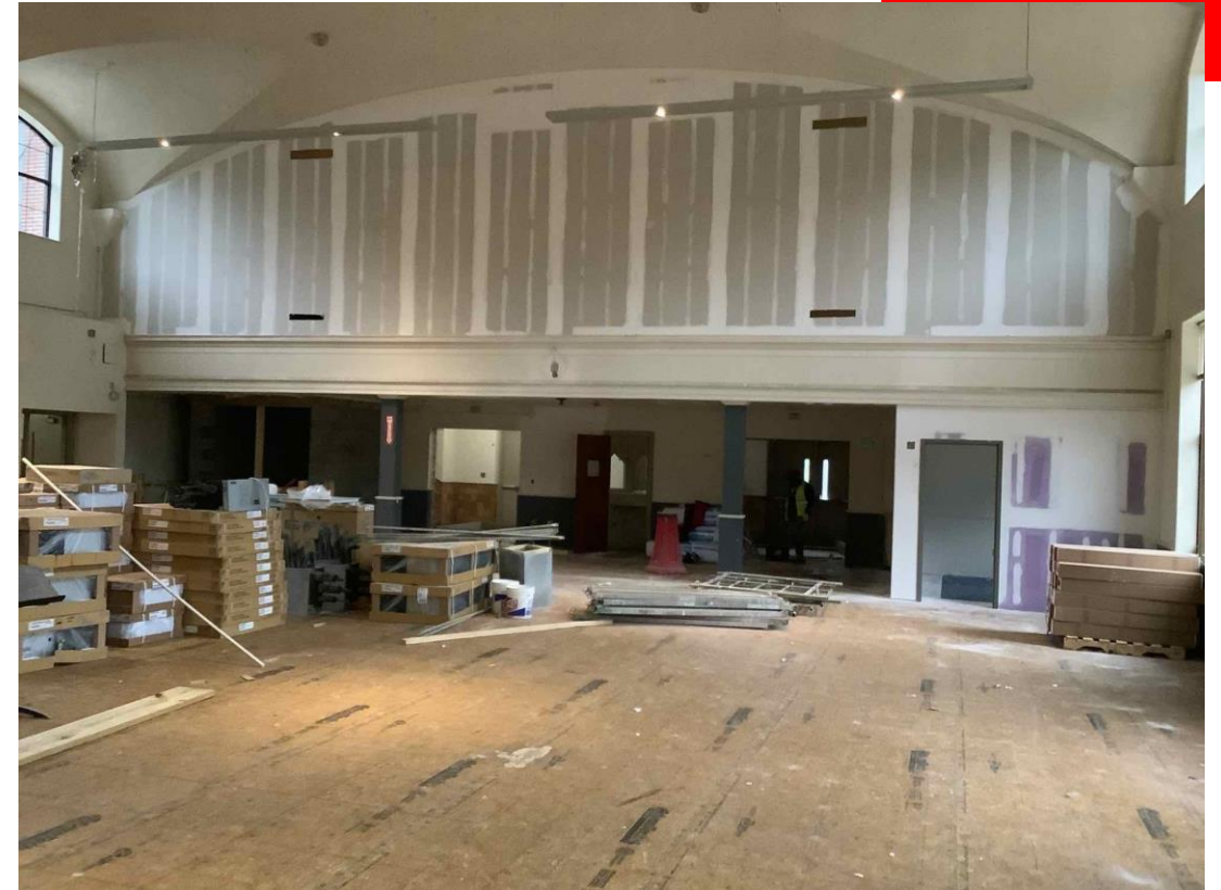
Interior framing and drywall at auditorium
